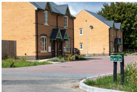
Photo 2 Entrance to the development
