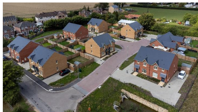
Photo 1 Hawes Lane Rural Exception Site
