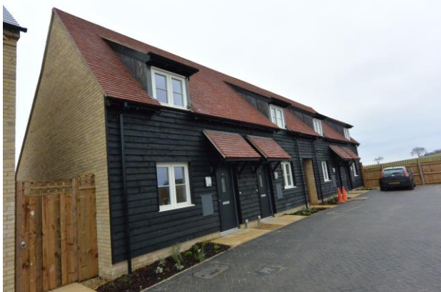
A 'barn-style' building incorporating 4x1 bed houses
