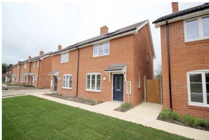
The scheme from the front, facing onto Whittlesford Road
